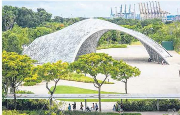
The Future of Us Pavilion by the Singapore University of Technology and Design, one of nine Design of the Year award winners, became a permanent landmark at Gardens by the Bay last year and plays host to festivals and other events. PHOTO: KOH SEE KIAT/ORDINARY STUDIOS
